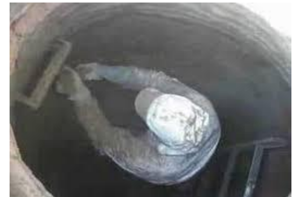
MANHOLE REHAB Cementitious Grouting
