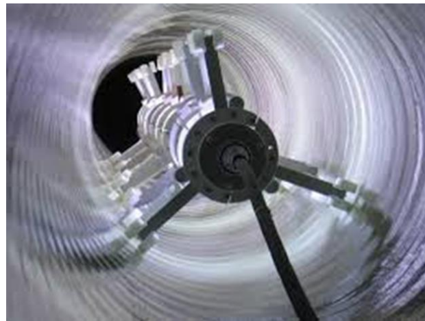
UV light Curing inside pipe Step 4 ( 3-6 hours, MH to MH)
