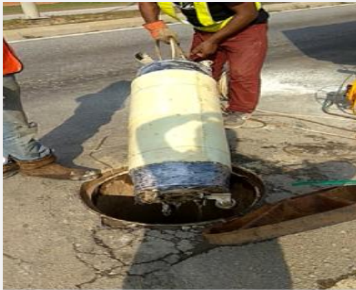
Move the packer down to the point of repair
