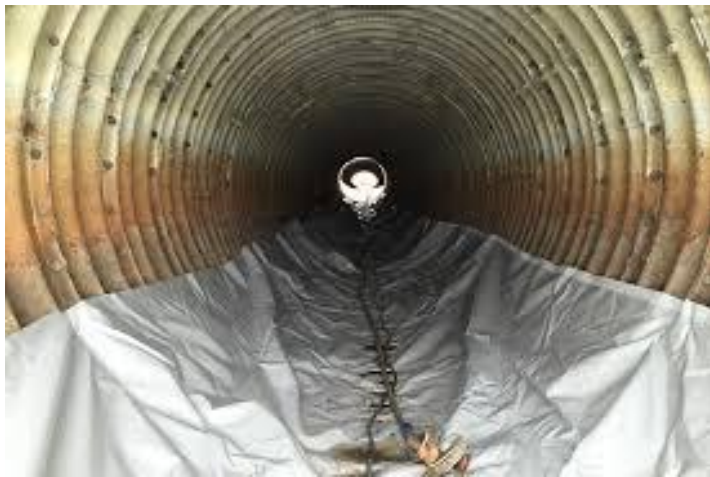
Liner insertion into pipe Step 2
