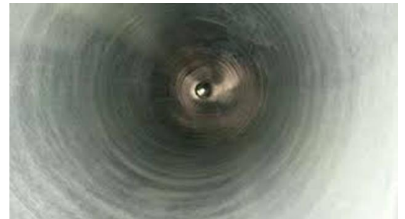
Step 5 - Finished curing inside pipe
