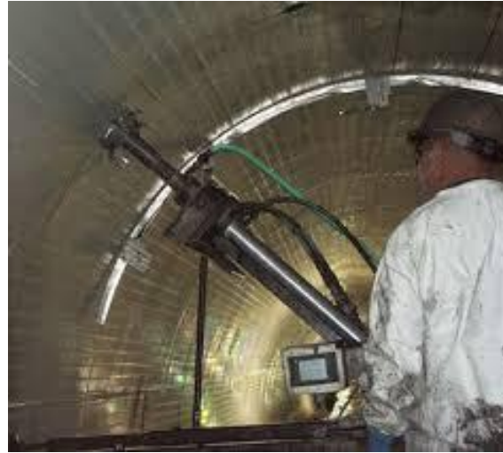
GiPP Injection Grouting 900/1200/1500 1800mm
