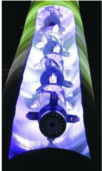
CIPP UV Curing 450mm
