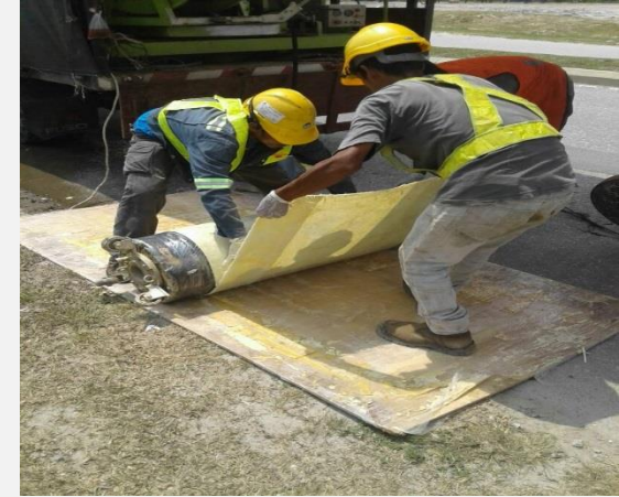
Wrap the impregnated fiberglass mat around the packer
