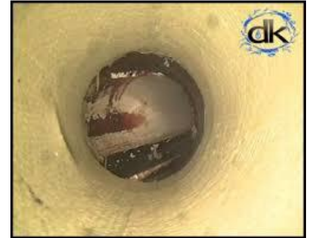
Step 5, Finished Cured Patch
