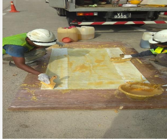
Pour & Spread the Silicate Resin uniformly with the hand spatula
